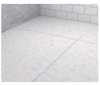
**Preparations for mounting**The exact course of the OKA-T trunking is measured and specified by tensioning a cord. Trunking branches are also marked on the raw
