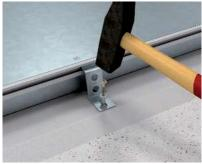
**Trunking fixing**Fix the aligned trunking section to the floor using the fixing bracket.
